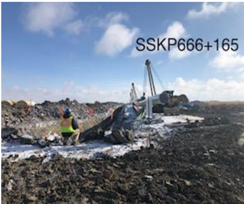
Lowering at SF75 East
