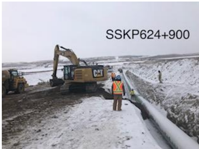
Backfill bellhole Chapleau Lake East
