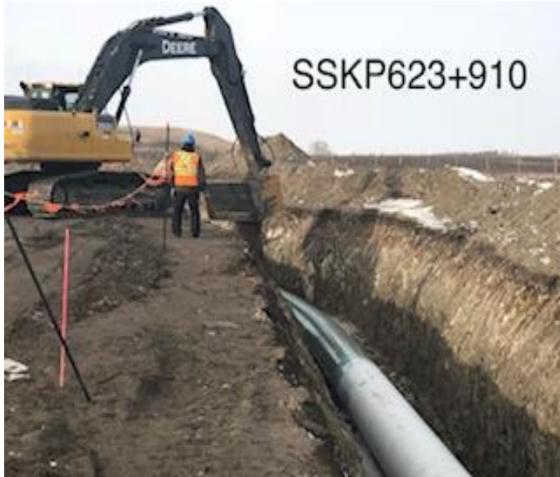
Shading in mainline ditch rock removal bucket
