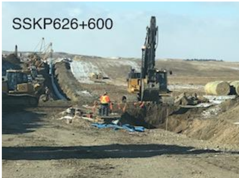
Lowered in gunite section at SF53 East
